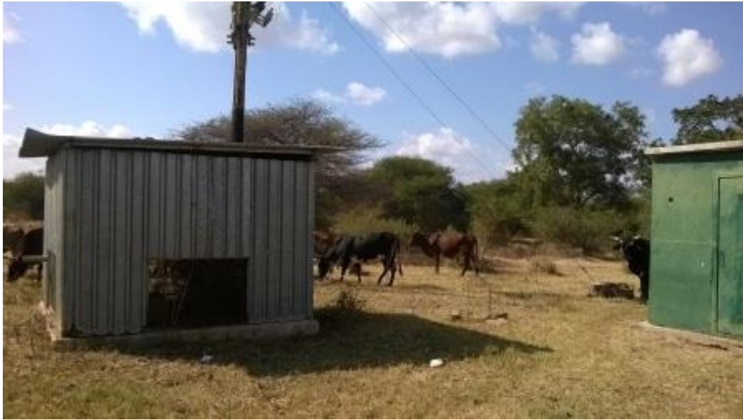
Figure 6.6 Community boreholes enclosed and locked away in order to prevent vandalism and misuse of the resource.
