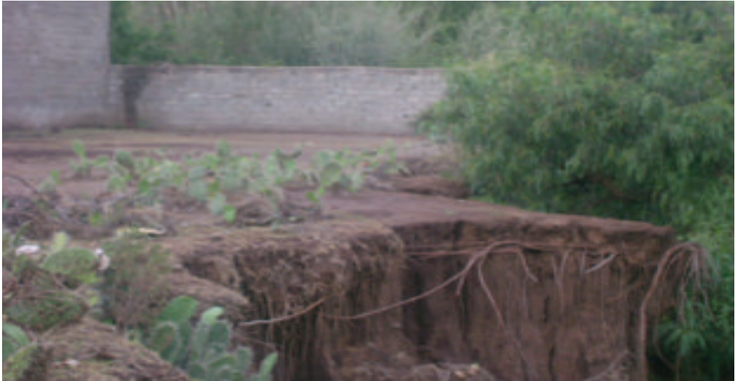
Figure 4. One of the huge gullies found within the City (2009)
