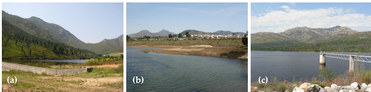
Figure 2-3. Overview of the three completed larger dams in the Langkloof valley. a) The Wabooms River dam, b) the Louterwater dam, and c) Haarlem dam
