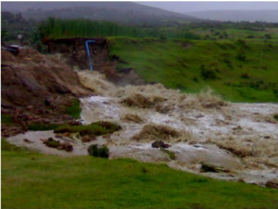
a. Dike burst after 2006 floods (1)
