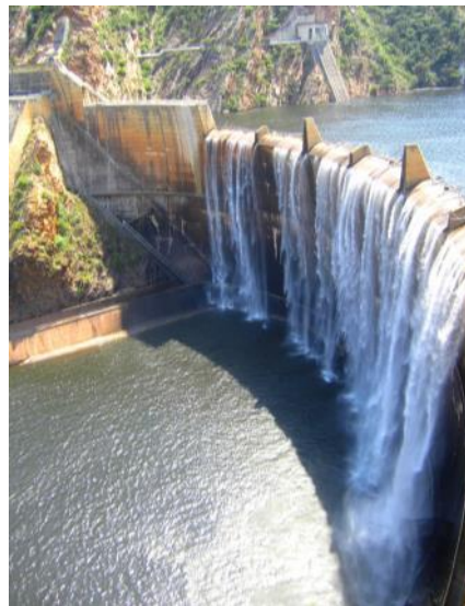
Figure 31: The Kouga dam is the biggest storage infrastructure in the catchment (around 400 hectares) (Photo: author)
