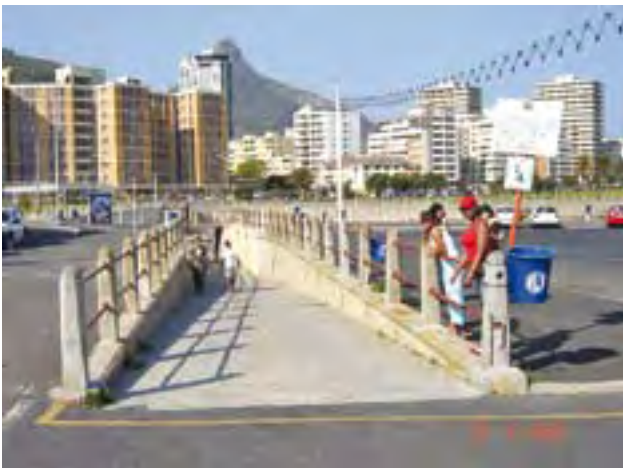
Above: This slipway at Three Anchor Bay does not meet the permit requirements, as there is no access control in place
