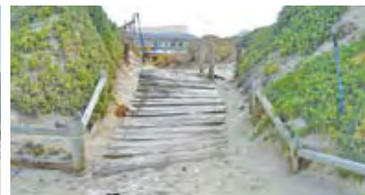
Chain Boardwalks at Fish Hoek Beach can be lifted as the Dune System grows
