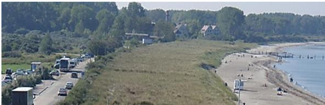
Figure 7.7: Examples of vegetated dikes (Germany)
