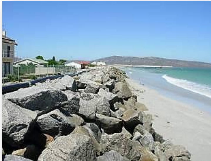
Figure 7.6: Example of a rock revetment protecting houses (South Africa)
