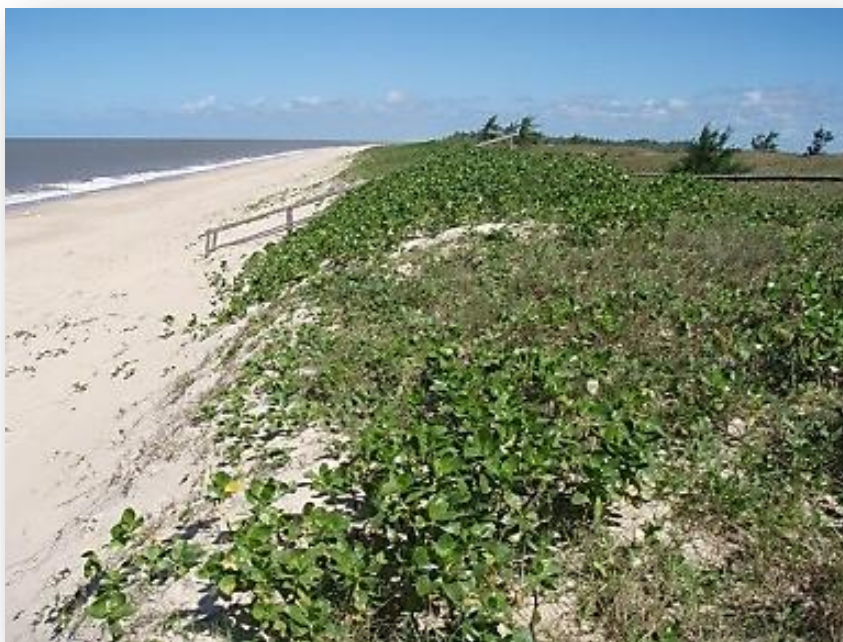
Figure 7.4: Example of a vegetated dune at Beira with sufficient volume and height to protect landwards areas from storm erosion or coastal flooding.
