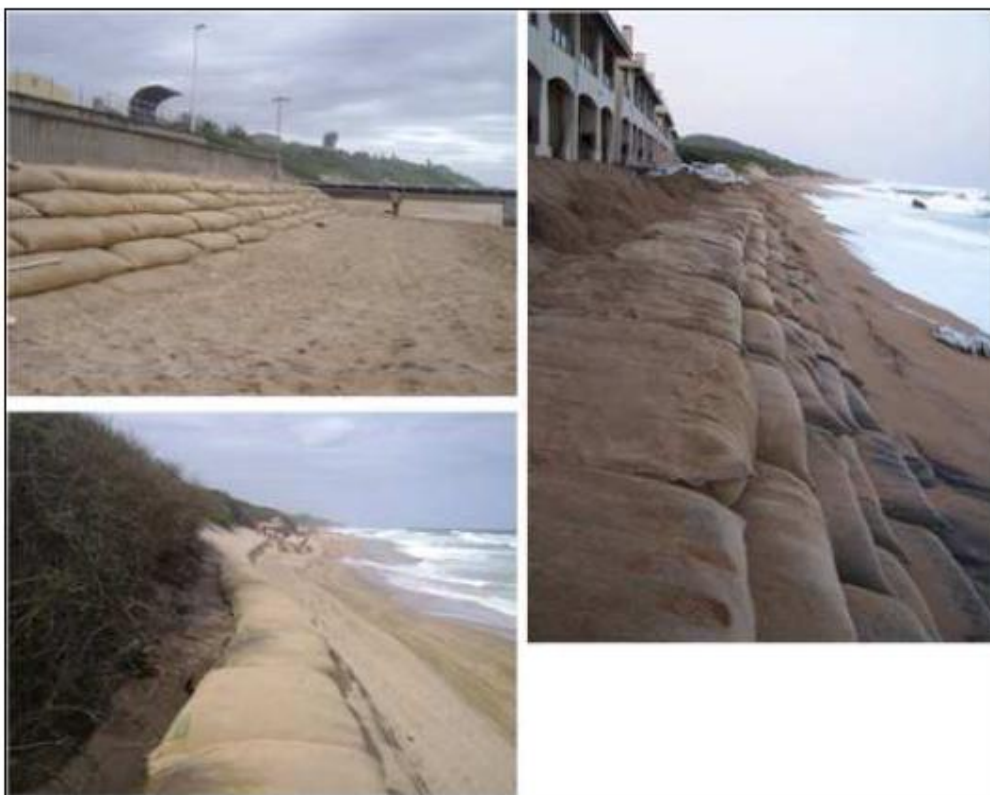
Figure 7.15: Examples of geotextile (sand bag) revetments (Kwazulu-Natal, South Africa)
